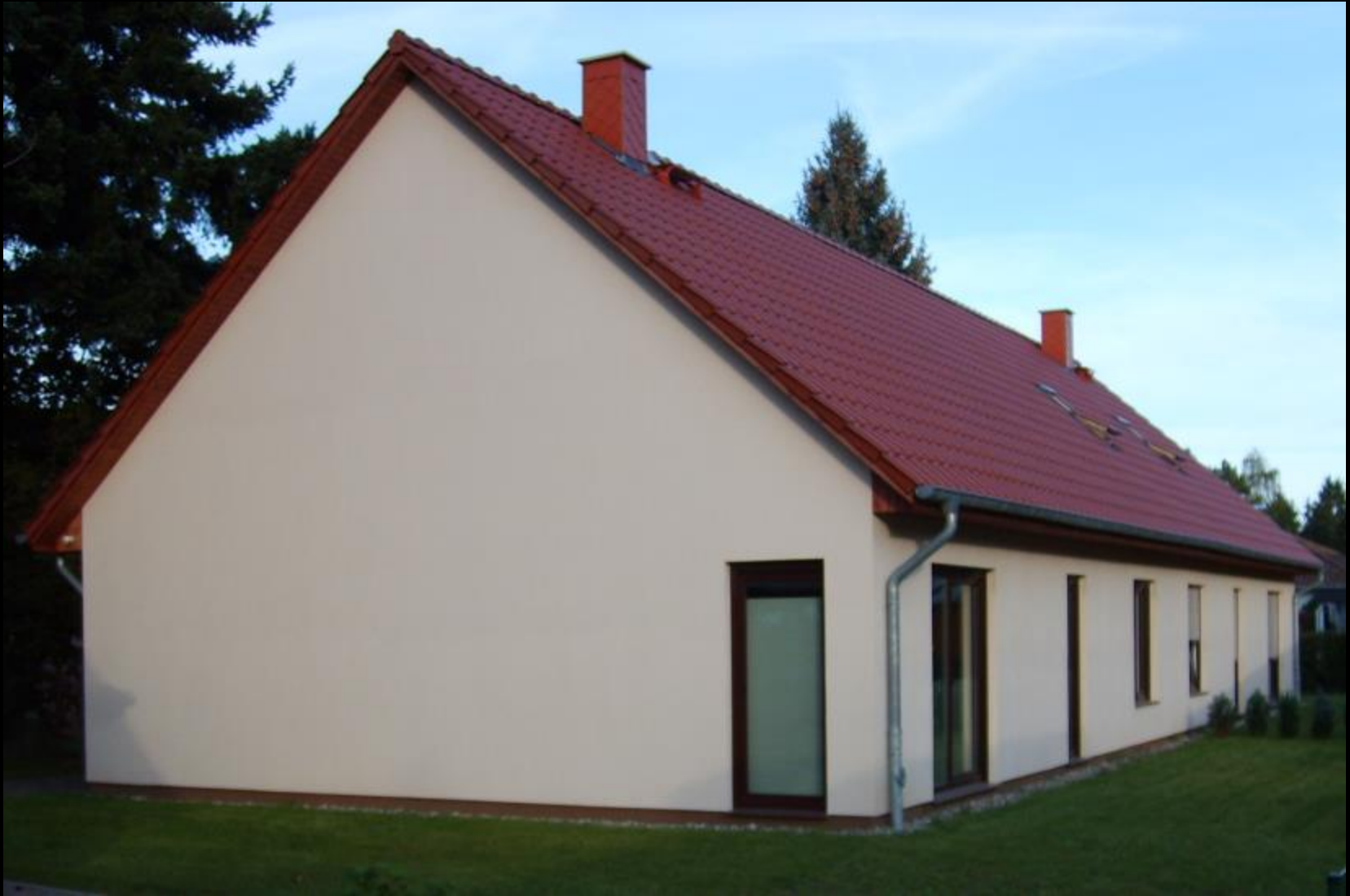
Typical german Passivhaus
